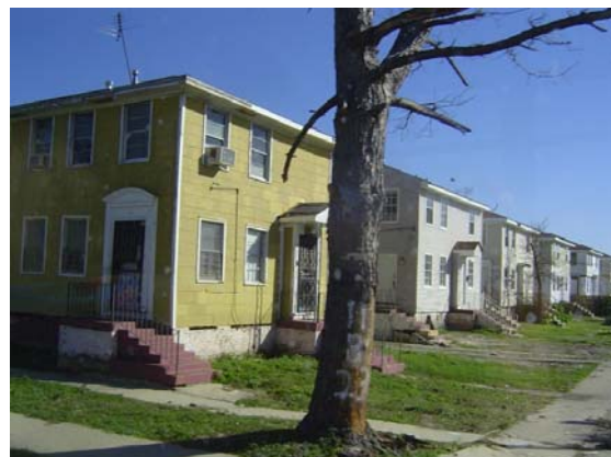
A residential street destroyed by flood
